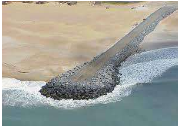
Slika 23 – Prikaz nasutog pera ( https://www.researchgate.net/figure/One-of-the-six-groynes-along-Keta-shoreline-source-Google-map_fig2_256756000 )
