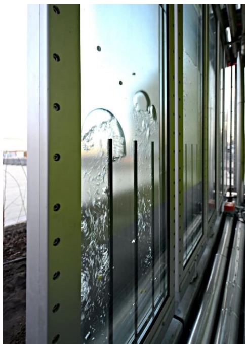
Slika 94: staklene fasadni bio-paneli koji su ugrađeni na zgradi u Hamburgu, (izvor: https://www.nytimes.com/2013/04/25/business/energy-environment/german-building-uses-algae-for-heating-and-cooling.html )
