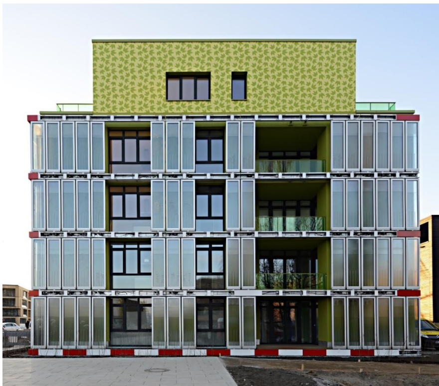
Slika 93: izvedena zgrada u Hamburgu koja koristi tehnologiju bio-panela na fasadama, (izvor: https://www.nytimes.com/2013/04/25/business/energy-environment/german-building-uses-algae-for-heating-and-cooling.html )
