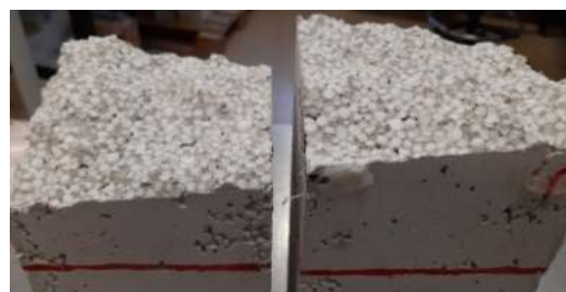
b) Failure surface
