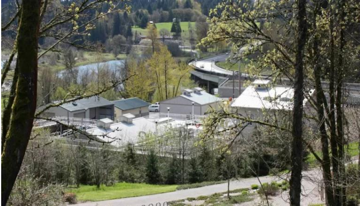
Slika 30. Pogled na UPOV La Center, Washington, SAD (The MBR site)
