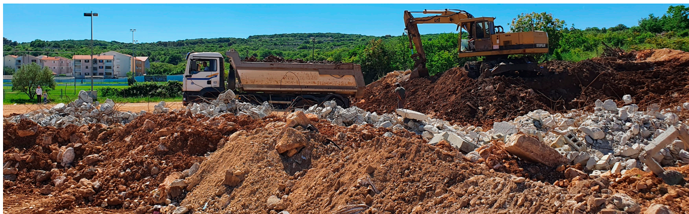
Figure 6. View of the observed construction site (private album of the first author).
