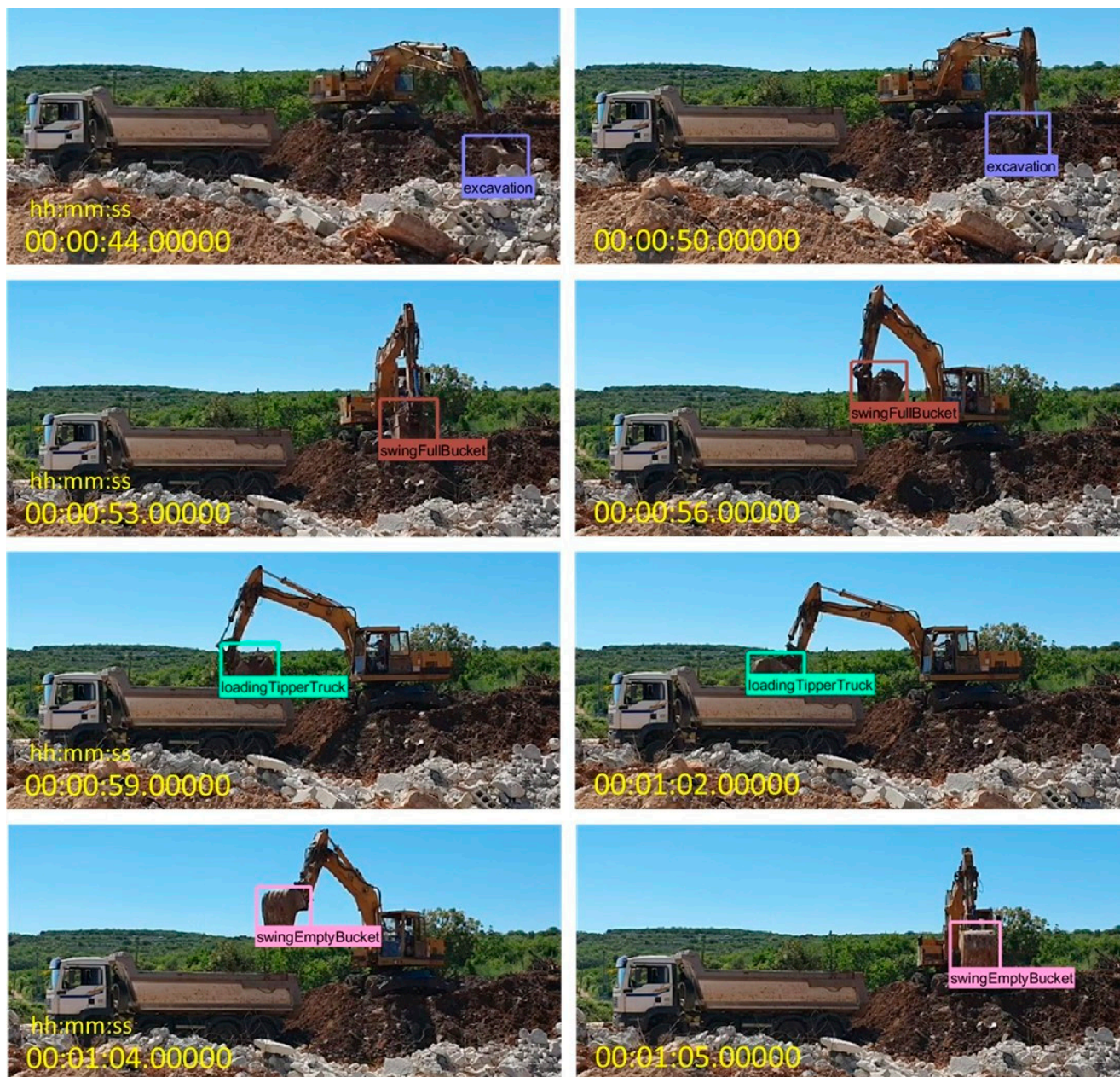
Figure 7. Examples of inserted labels for excavator working operations from the first video of loading (image created using MATLAB by the first author).
