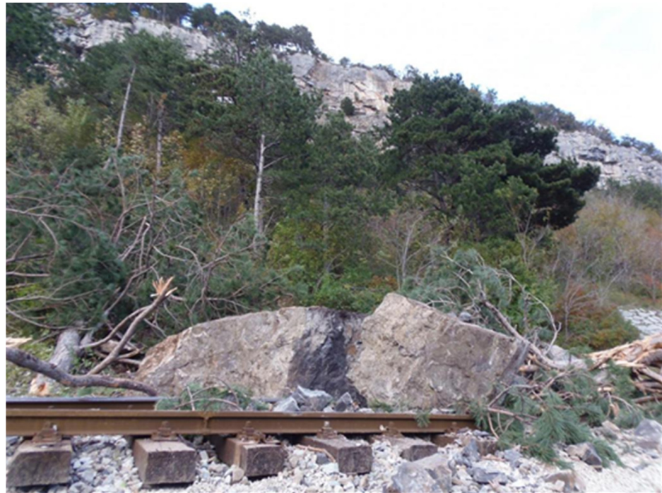
Figure 5. Photo of the rockfall originating from the Raspadalica Cliff on 16 December 2013.
