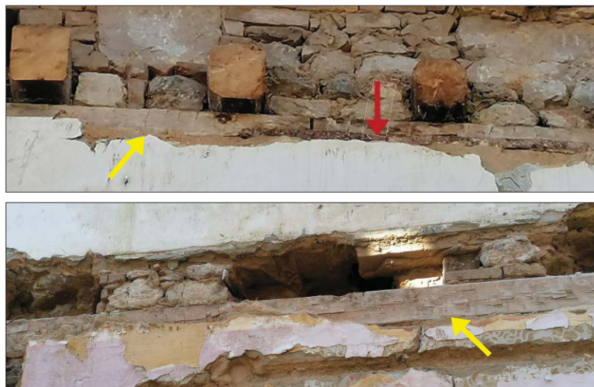
Figure 5. Timber ring beams at the floor levels.
