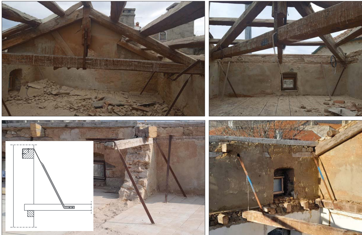
Figure 8. a) Diagonal wall-to-floor iron ties.
