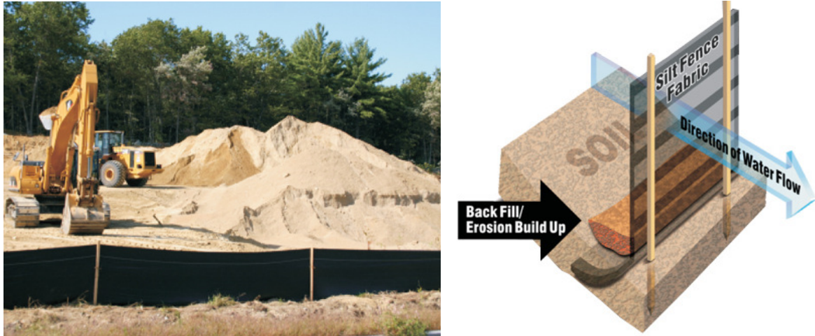
Figure 58: Silt fences ( http://www.grip-rite.com/ )
