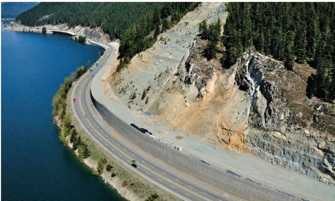
Slika 6. Kolnički nasip ( https://reinforcedearth.com )
