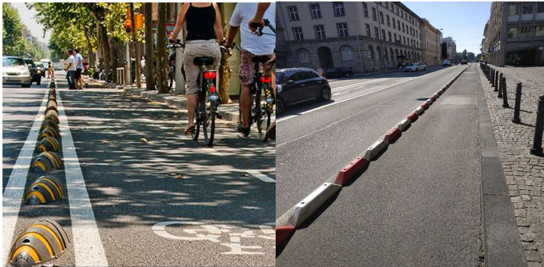
Figure 43: Protected cycle lane in the carriageway level [13]
