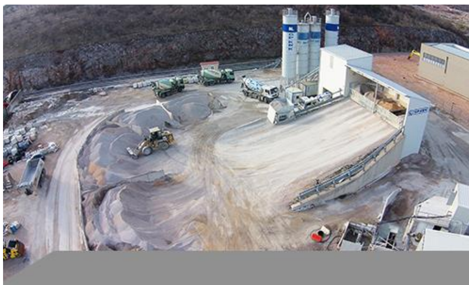
Slika 27: Betonara Kukuljanovo - GP Krk
