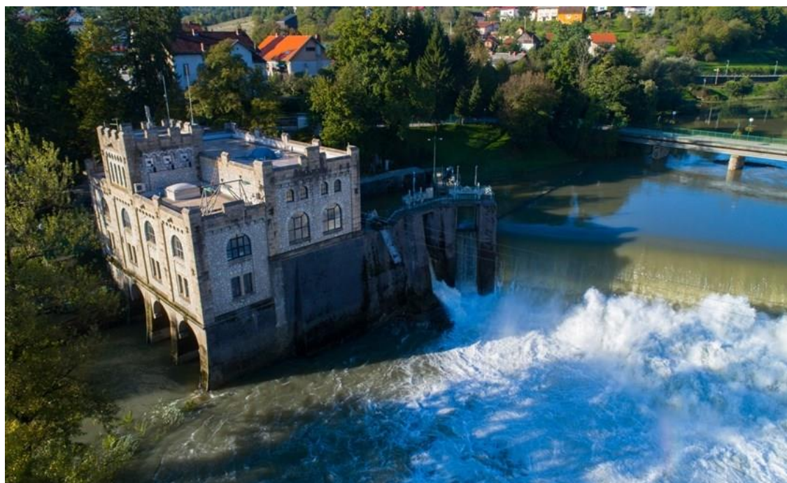
Slika 2.18. HE Ozalj I ( https://www.hep.hr/proizvodnja/hidroelektrane-1528/pp-he-zapad/he-ozalj-1-i-2/1544 )
