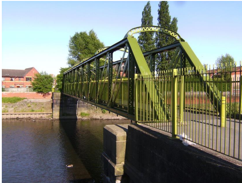
Slika 12. Izgled mosta danas, Prattova rešetka ( https://en.wikipedia.org/wiki/File:Broughton_bridge.jpg )
