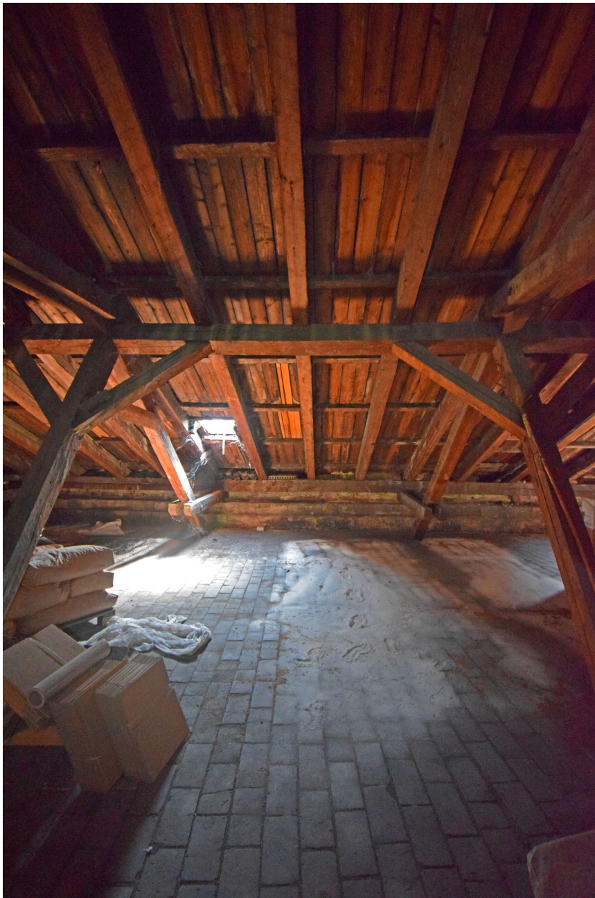
Figure 15. Tobacco Factory H-building, roof details (Marko Franković, 2018).
