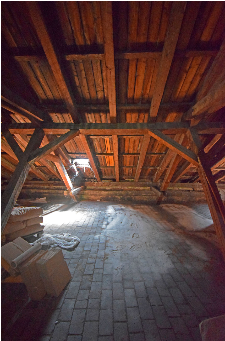
Figure 15. Tobacco Factory H-building, roof details (Marko Franković, 2018).
