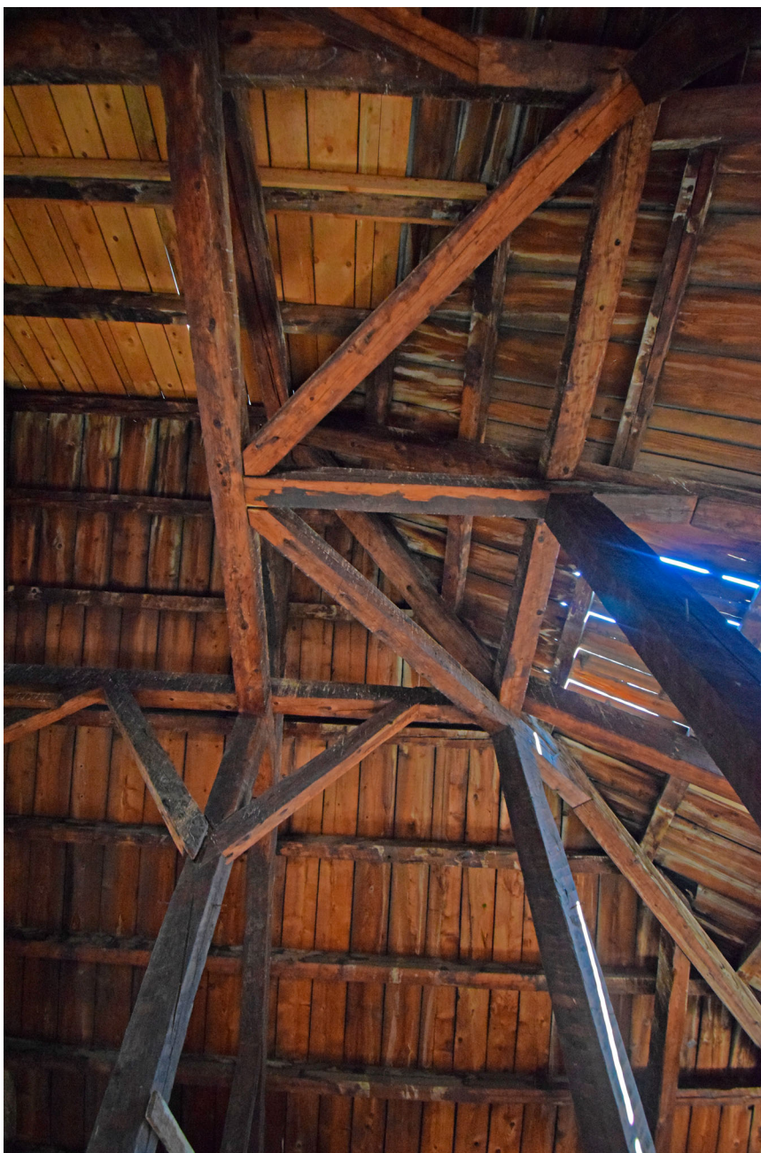
Figure 9. Tobacco Factory T-building, roof structure detail (Marko Franković, 2018).
