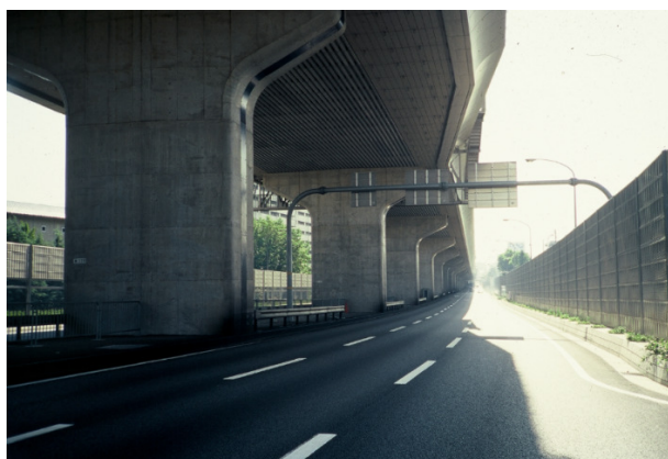
Figure 3. The Fukae section Kobe Route expressway after retrofit implementing measured presented in Fig. 6b (Copyright: M. Čaušević)
