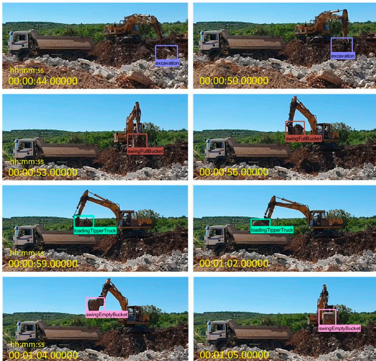
Figure 7. Examples of inserted labels for excavator working operations from the first video of loading (image created using MATLAB by the first author).
