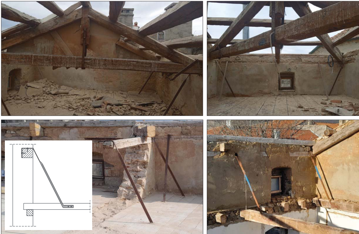
Figure 8. a) Diagonal wall-to-floor iron ties.
