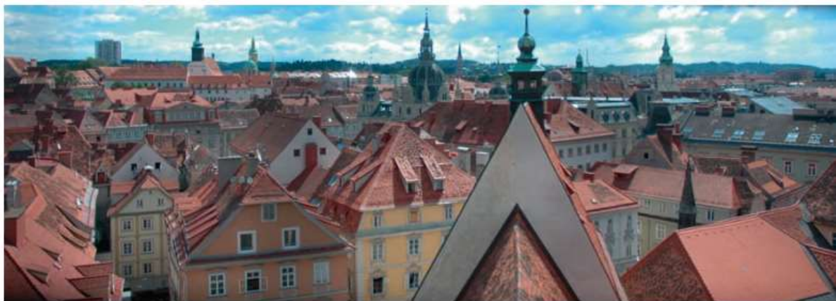
Figure 1.3. View on the roofs in Graz, old town [16]
