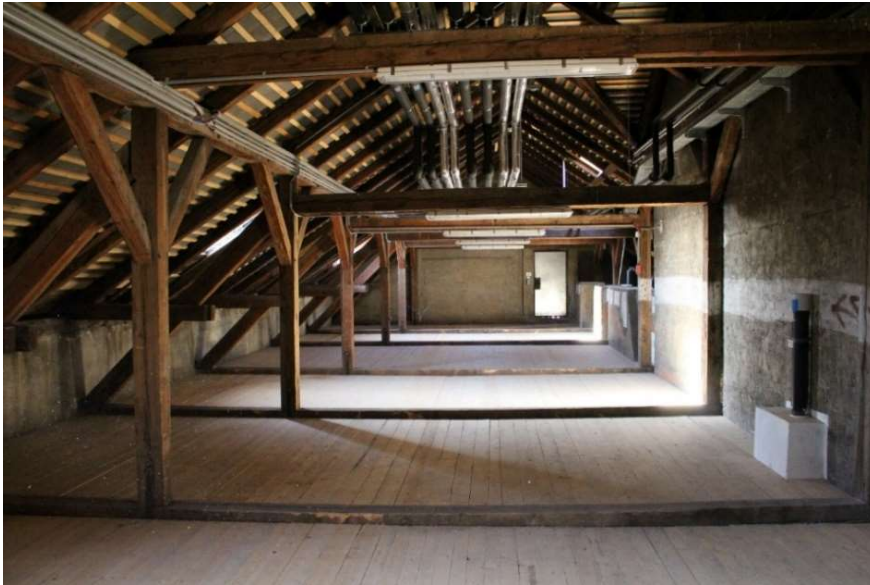
Figure 2.4. View on the roof structure in room 2
