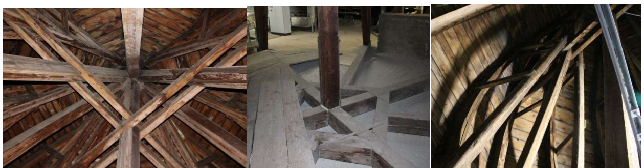
Figure 2.13. left: View on the dome spike; centre: Tie beams, secondary tie beams and central post; right: Main rafter unit
