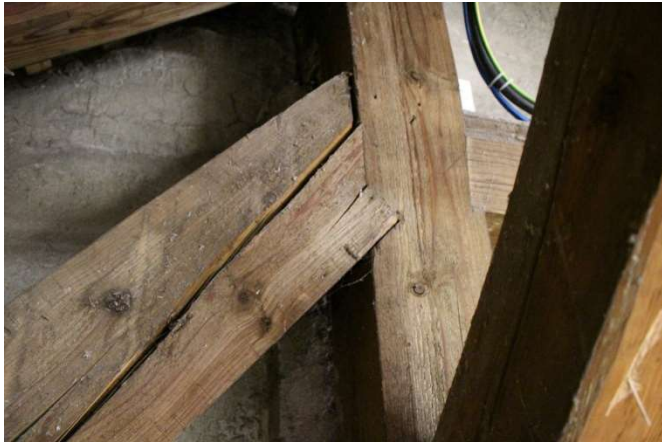
Figure 2.25. Connection Brace to Queen post
