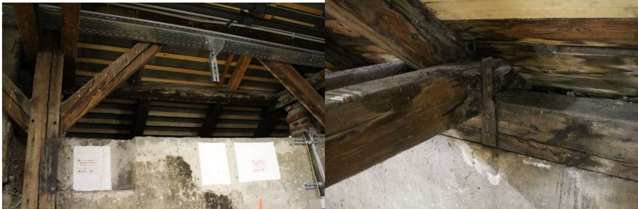
Figure 4.4. left: The white colour of the transversal beams and dark stripes on the knee brace; right: Sap fungi and wood oxidation
