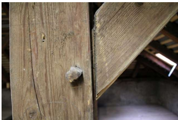
Figure 2.27. Detailed view on tenon and wooden peg
