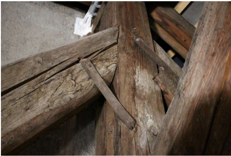
Figure 2.7. Connection brace - post in axis 13 and 14
