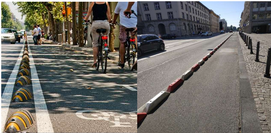
Figure 43: Protected cycle lane in the carriageway level [13]
