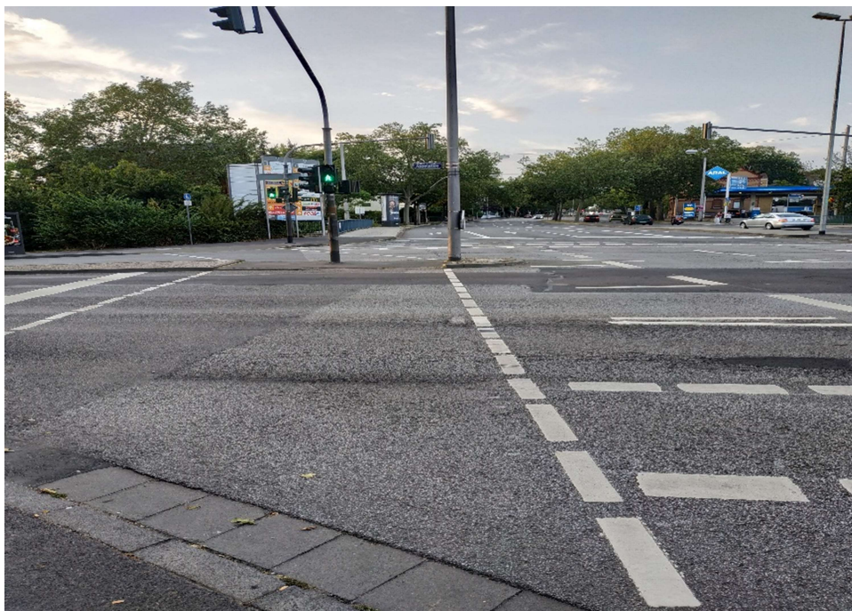
Figure 17: Cyclist crossing adjacent to the pedestrian crossing
