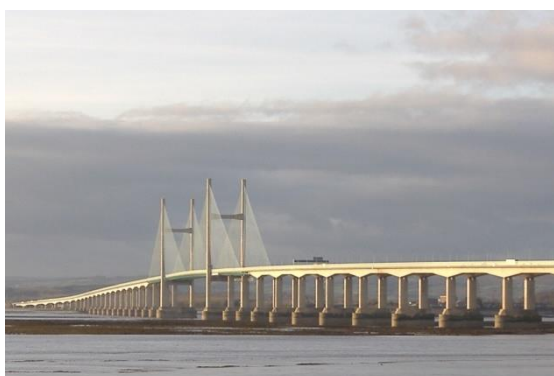
Slika 39: Second Severn Bridge, UK [38]
