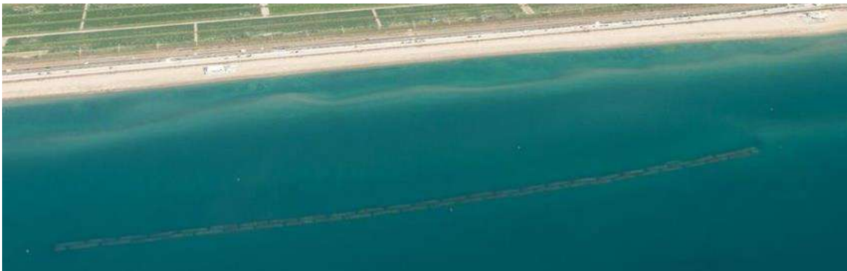
Slika 22. Potopljeni lukobran ( https://www.researchgate.net/figure/Aerial-view-of-the-installed-submerged-breakwater-with-encapsulated-sand-filled-elements_fig3_321056403 )
