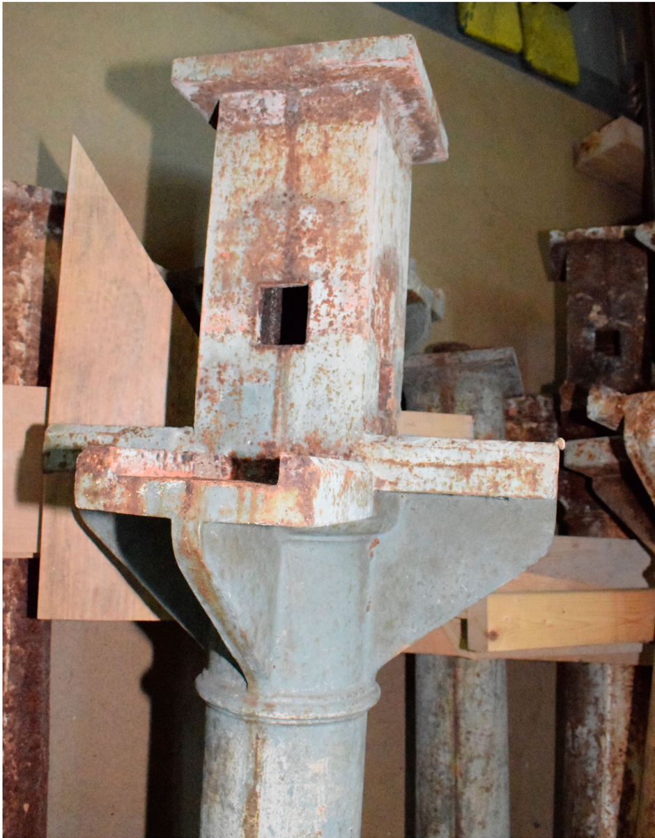
Figure 18. Tobacco drying facility, detail of column (Marko Franković, 2019).
