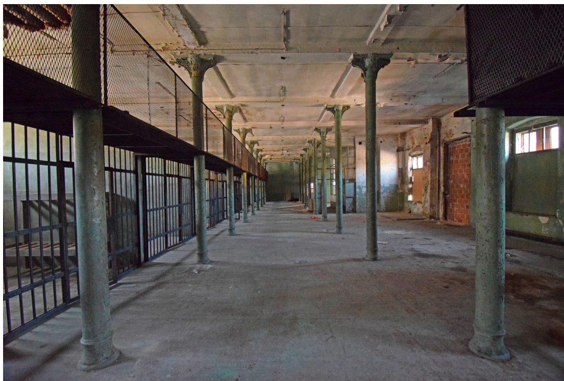
Figure 6. Tobacco Factory T-building, first-floor skeletal structure (Marko Franković, 2018).
