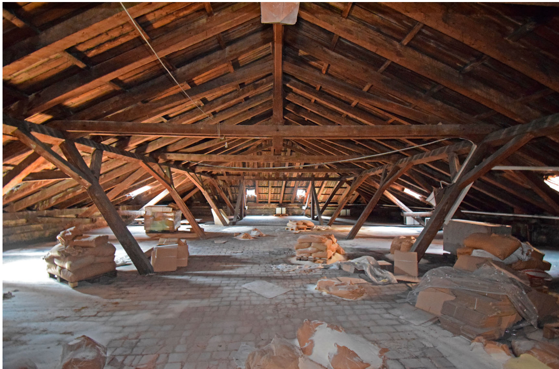
Figure 14. Tobacco Factory H-building, roof structure (Marko Franković, 2018).
