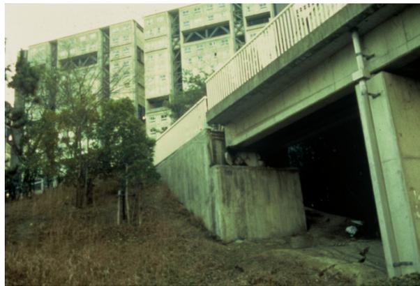
Figure 5. Sliding displacement of a bearing device of bridge superstructure and inclination (damage) of reinforced concrete pier wall, Ashya Seaside Village in Kobe, the 1995 Kobe earthquake;
