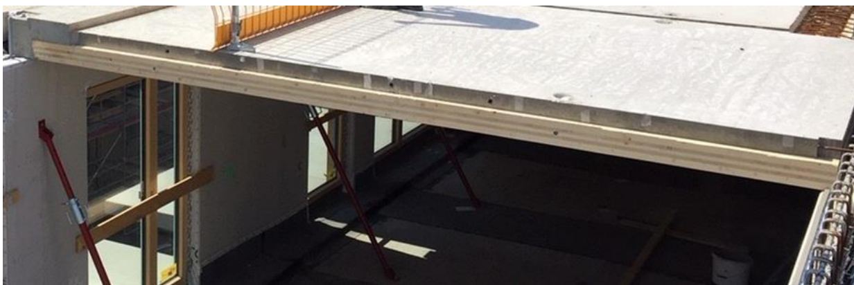
c) Predgotovljena TCC stropna ploča velikog raspona (dimenzije 10 x 3 m) (izvor: https://www.mm-holz.com/en/products/timber-concrete-composite-element )
