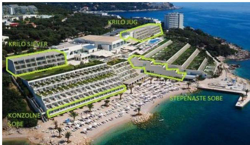
Figure 12. Plan of added parts of the hotel accommodation tract. D. Sošić: Reconstruction of Hotel President in Dubrovnik in 2013, Master's thesis, University of Rijeka, Faculty of Civil Engineering, Rijeka, 2020.
