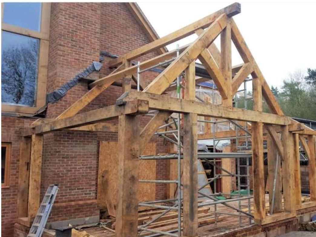
Slika 12: Skeletni sustav (izvor: https://www.timber-frame-suppliers.co.uk/about-timber-frame/ , 16.06.2024.)
