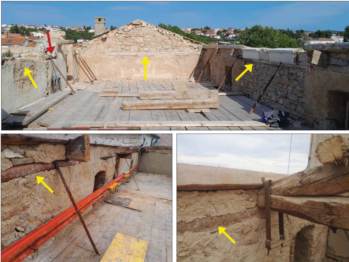
Figure 4. Timber ring beams at the roof level.
