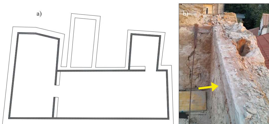
Figure 3. Timber ring beams at the roof level: a) Ground plan; b) Detail.
