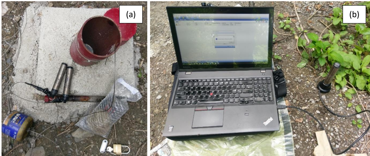
Figure 12: Collection of continuous groundwater pressure measurements at the B2 location: a) Rugged TROLL 100 Data Logger and BaroTROLL Data Logger (In-Situ Inc.), and b) TROLL Docking Station for periodical download of the recorded data with the Win-Situ 5 software (In-Situ Inc.).
