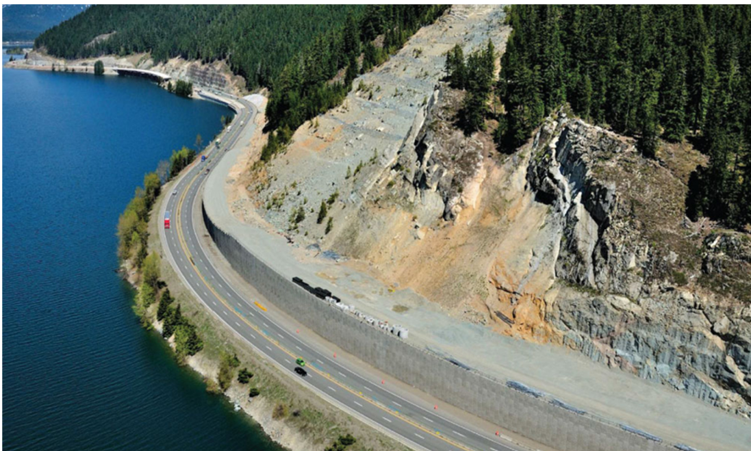
Slika 6. Kolnički nasip ( https://reinforcedearth.com )
