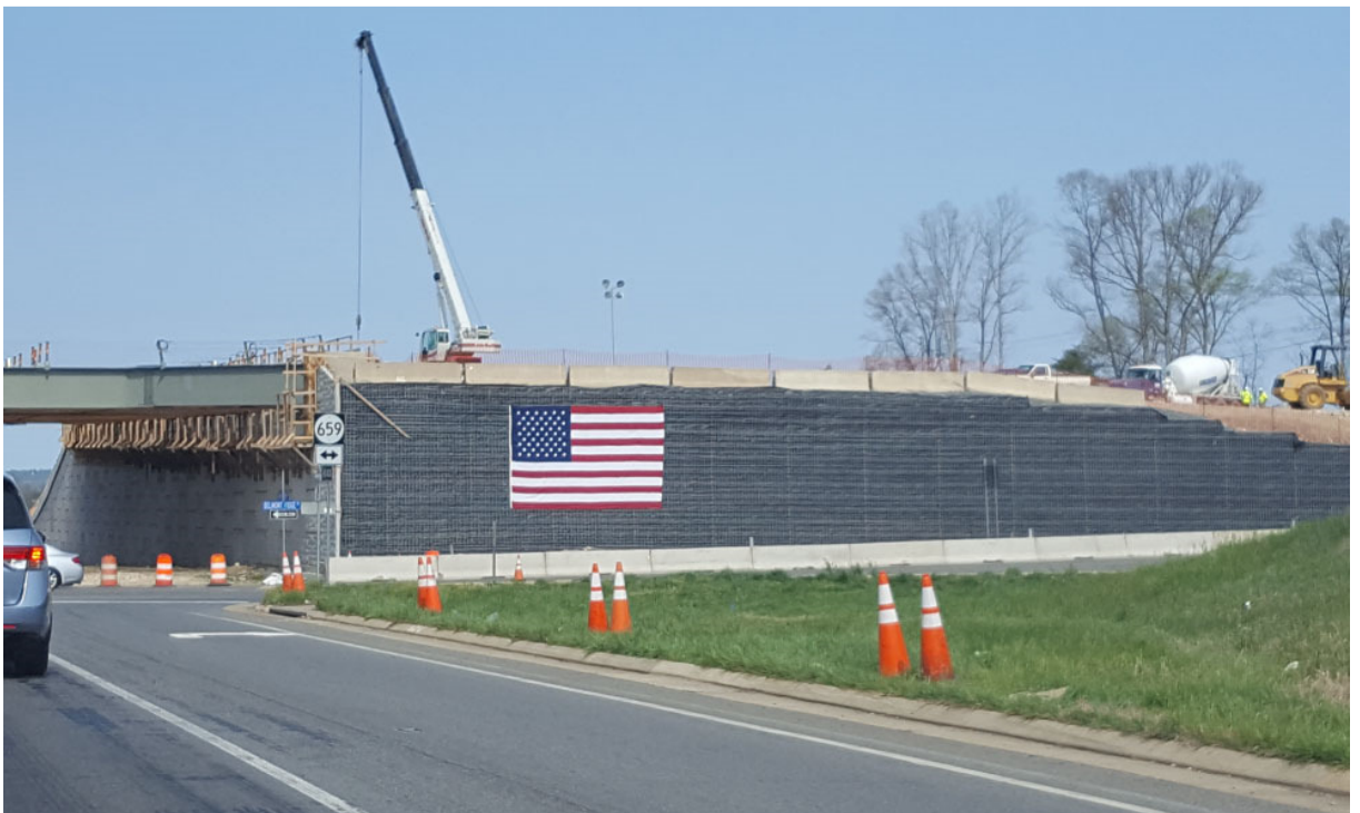
Slika 14. Privremeni potporni zid ( https://reinforcedearth.com )
