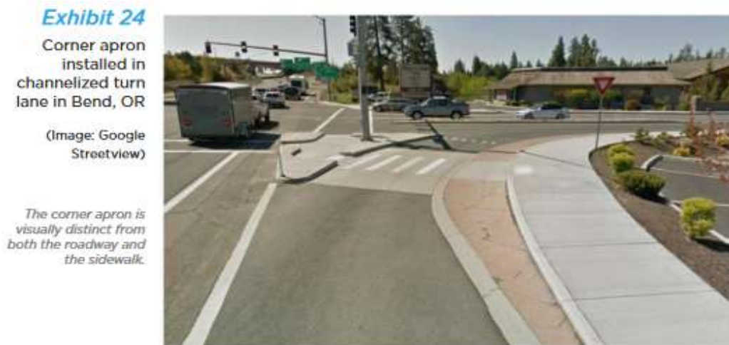
Figure 48: Example of a mountable corner apron [17]
